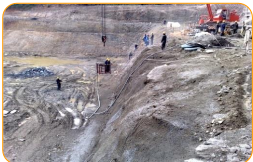
Shotcreting for power intake at 489.500 m depth
