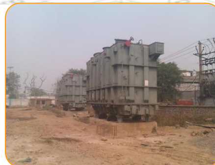
100MVA Transformer, EMCO
