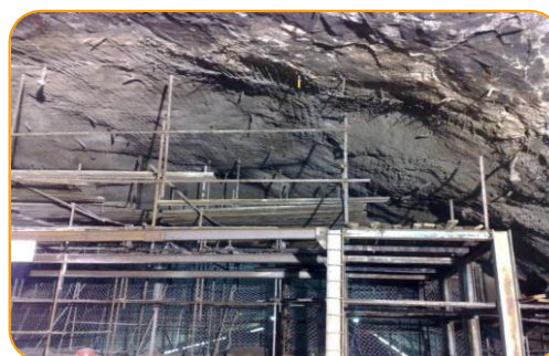
Shotcreting of crown at Extension Power House
