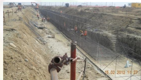
Cable Tunnel under construction
