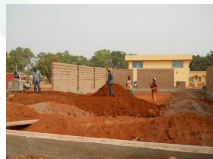
Sub-Station Foundation work in progress
