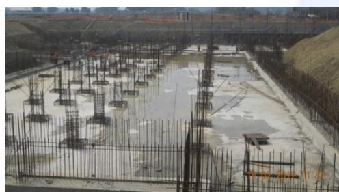
Raft for Load Block Sub station, Sinter Plant
