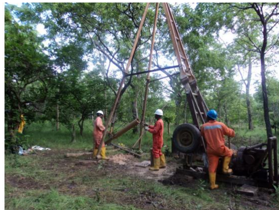
Borelog Data Collection at site by Geotech Agency
