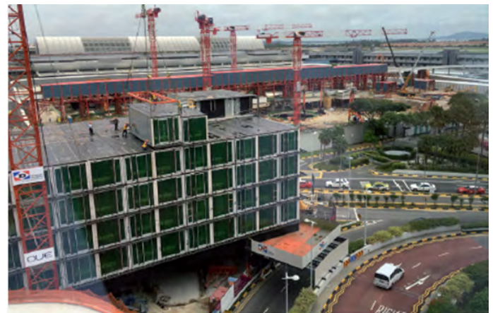
Figure 3: PPVC technique of construction in Singapore 2
