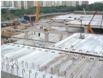
Fig. 3 R.C. Planks laid over partially precast joists
