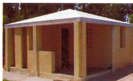
Fig.12 Un Reinforced Pyramidal Brick Roof
