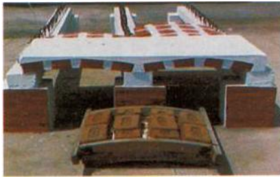
Fig. 7 Pre Fab Brick Arch Panel
