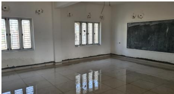
BALAPUR SCHOOL, HYDERABAD CONSTRUCTION WORK
