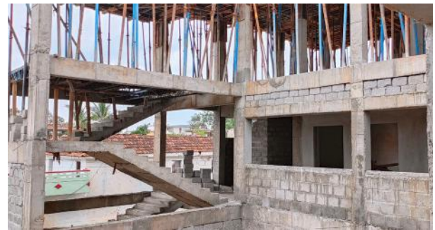
DEVARYANJAL SCHOOL CONSTRUCTION WORK
