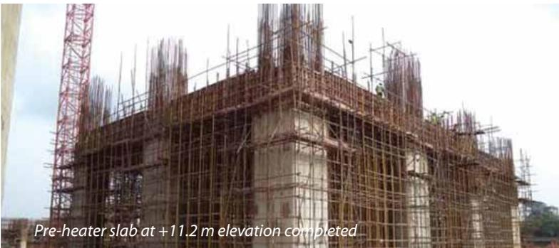
Pre-heater slab at +11.2 m elevation completed
