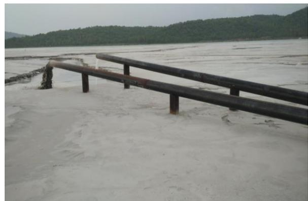
Figure 1. Existing ash pond with ash slurry filled up to the maximum ash fill level.
