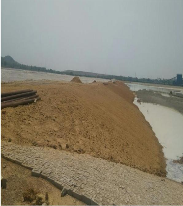
Figure 16: Construction of first stage raising of ash bund
