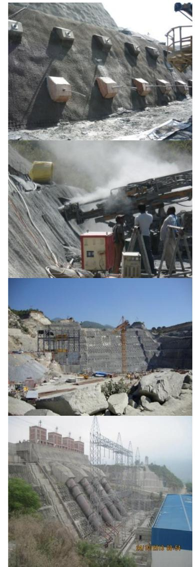
Slope stabilisation with prestressed anchors
