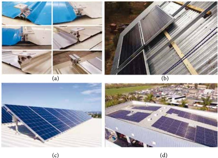
» **Figure 1** (a) Typical panel clamping detail; (b) Typical panel installation on steep slope; (c) Panels mounted on frames; (d) Panels mounted on low sloped roof
