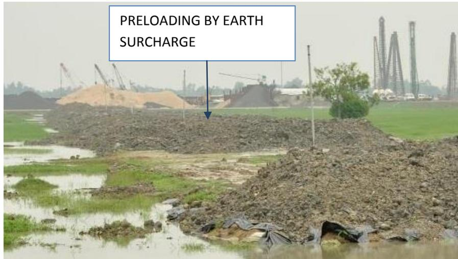
Fig – 2 Preloading by earth surcharge
