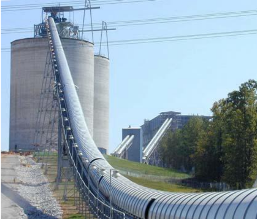
Fig. 6 Concrete silos for the coal storage.
