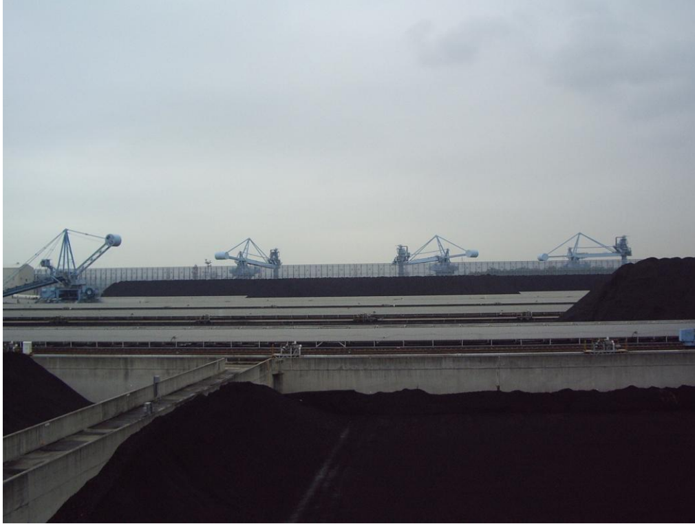
Fig. 5 Typical Wind barrier for the coal stockpile
