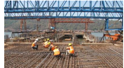
Main berth work in progress
