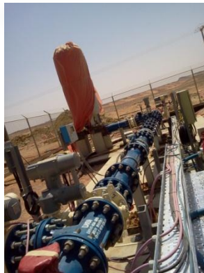
Commissioning Team assistance during pre-installation checks and Installation of Pump
