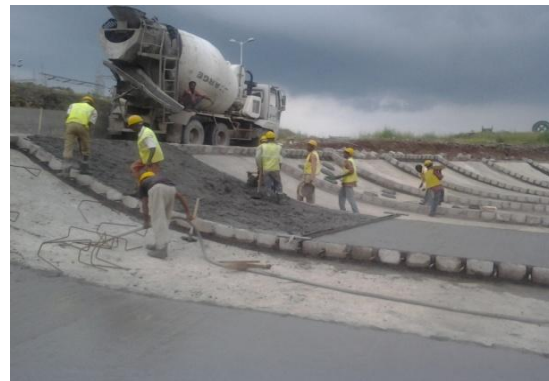
Construction of super-elevation in progress.
