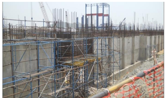
Construction of MSDS
