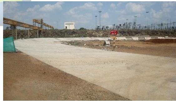
Construction of super-elevation in progress.
