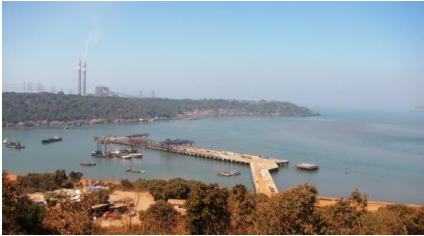
View of cargo jetty
