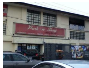
Supermarket at Harcourt
