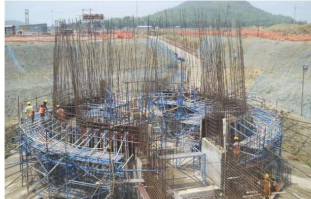
Reinforcement Fixing in progress for Chimney
