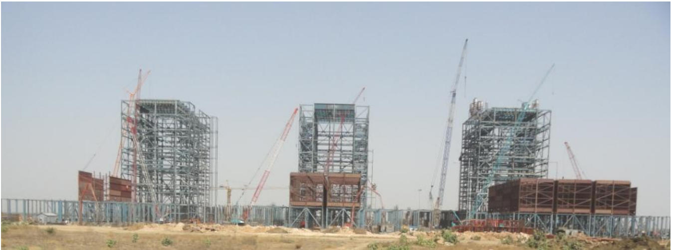
3x660 MW Boiler and ESP Structure
