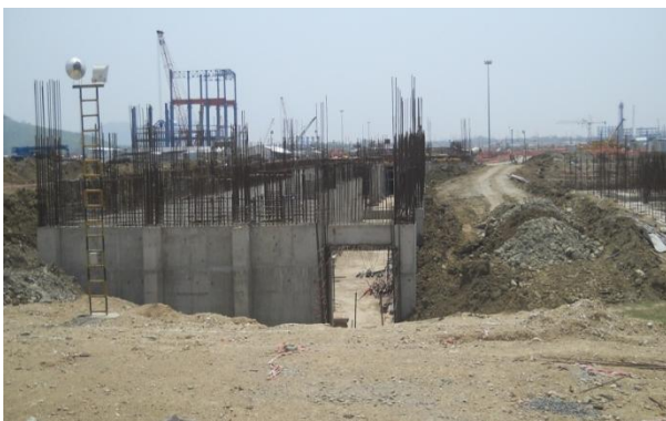
Construction of MRSS-220 kV
