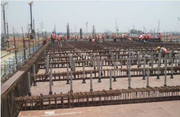
Nozzle Pipe Fixing in progress for Battery 2
