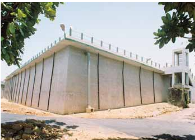
▲ Worli Water Reservoir, Mumbai
