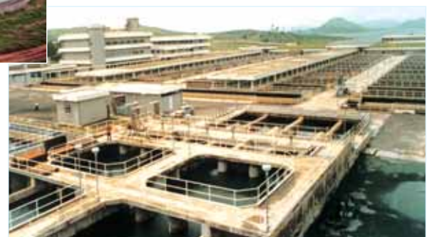
▲ Bhandup Water Treatment Plant, Mumbai
