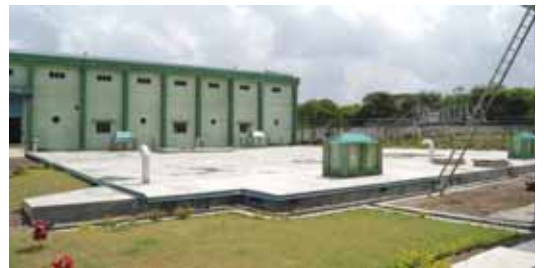
▲ Water Treatment Plant Reservoir, Nagpur
