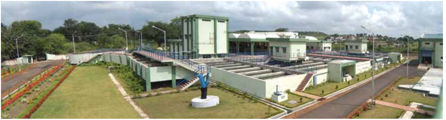
▲ Water Treatment Plant, Nagpur
