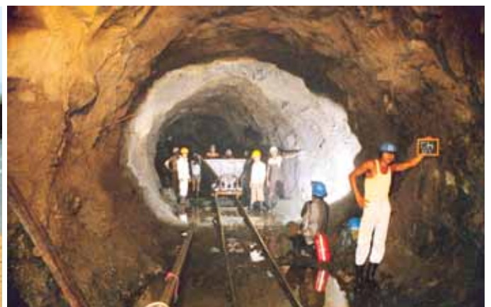
▲ Kasheli Water Supply Tunnel, Mumbai
