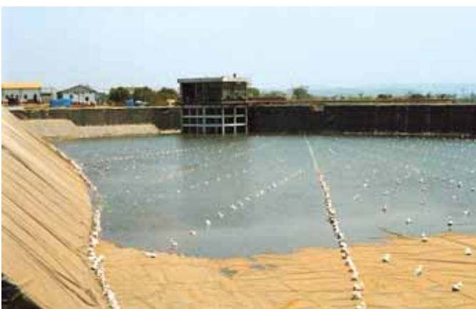
▲ Emergency Water Reservoir, Dabhol Power Plant
