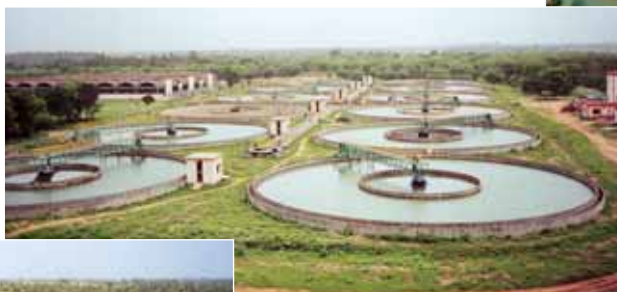
▲ Kotarpur Water Treatment Plant, Ahmedabad
