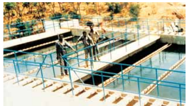
▲ Water Treatment Plant Filters, Lilongwe City, Malawi
