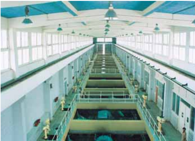
▼ Clear Water Pumping Station, Bhandup
