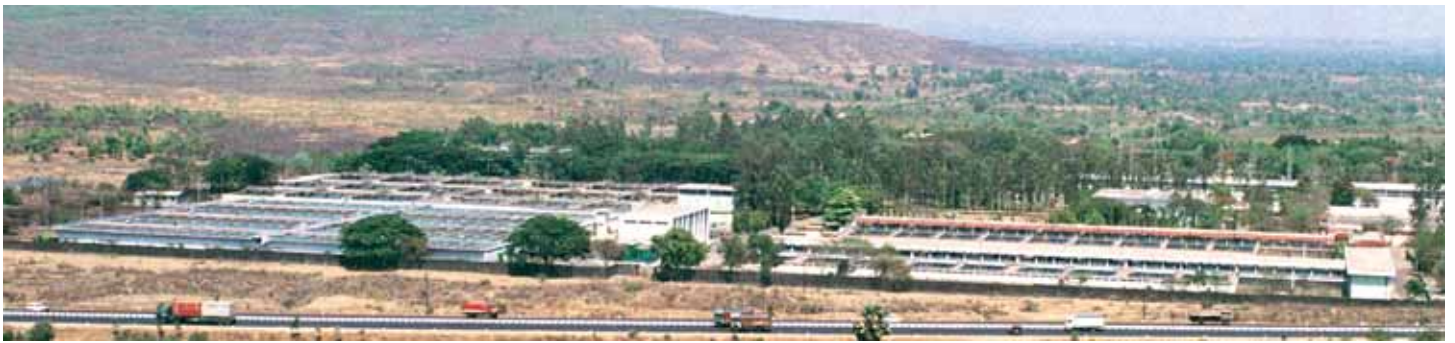
▲ Panjrapur Water Treatment Plant, Mumbai
