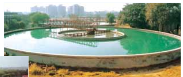
▲ Clarifloculator, Haidarpur Water Treatment Plant, New Delhi
