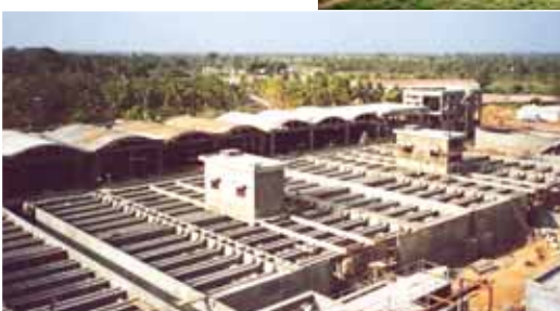
▲ T K Halli Water Treatment Plant, Bangalore
