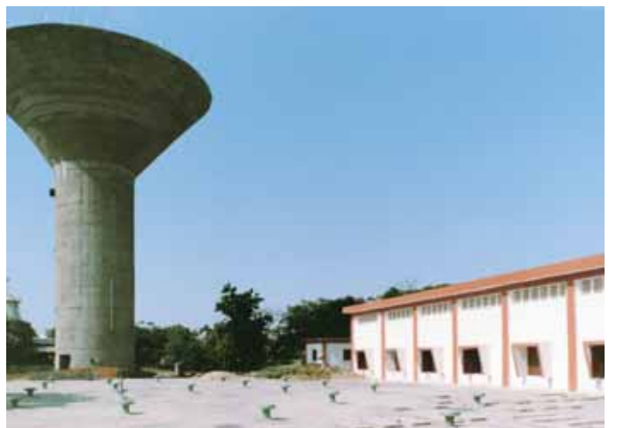
▲ Dhudheshwar Water Storage Tank, Ahmedabad
