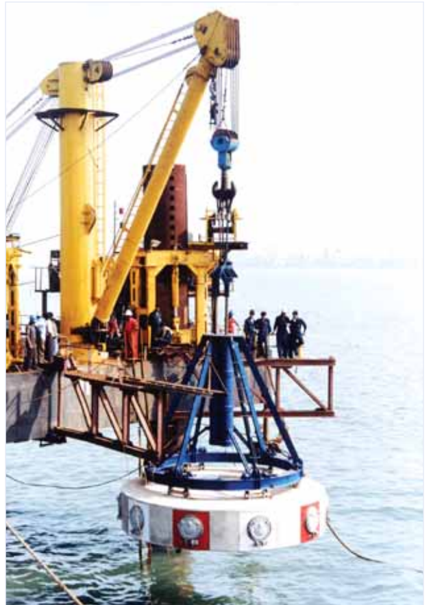
▲ Installation of Riser for Marine Outfall, Mumbai
