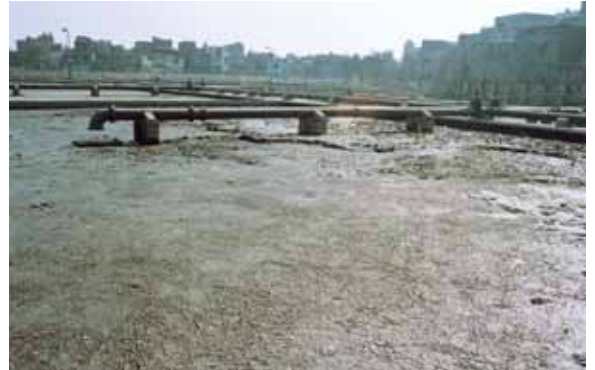
▲ Sludge Drying Beds, New Delhi
