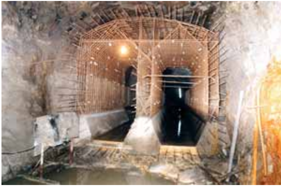
▲ Waste Water Conveyance RCC duct, Mumbai
