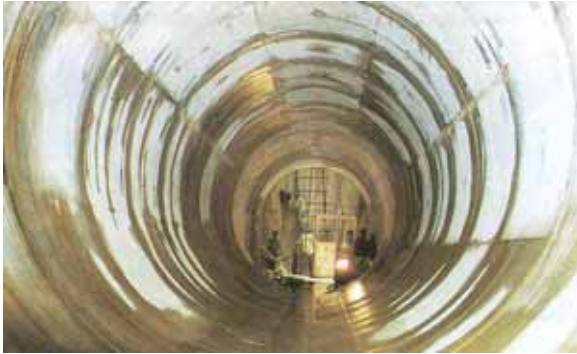
▲ Pre-cast RCC segmentally lined Waste Water Conveyance Tunnel, Mumbai
