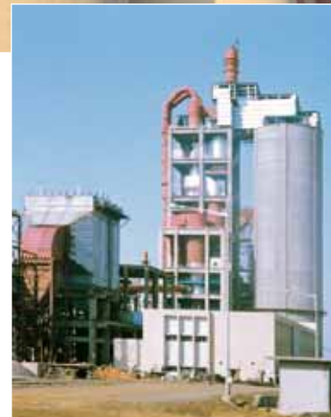
▲ Cement Plant, TISCO, Sonadih
