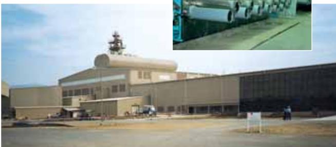
▲ Owens Corning's Fibre Glass Plant, Talaja
