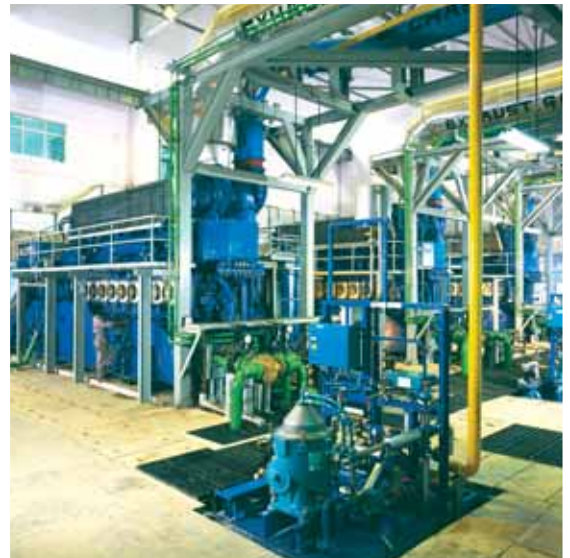
▲ 3 x 3 MW Diesel Generator Sets, ITPL, Bangalore
