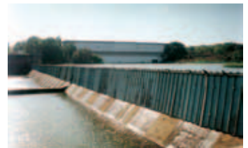
Pise Weir in raised position, Mumbai
