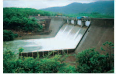
Kundli Pumping Scheme, Phase II
