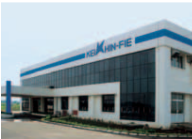
Carburetor Manufacturing Plant, Pune
