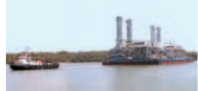
220 MW Barge Mounted CCPP, Tanir Bavi
