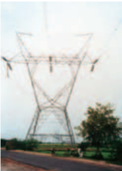
800 kV Anpara-Unnao Transmission Line
